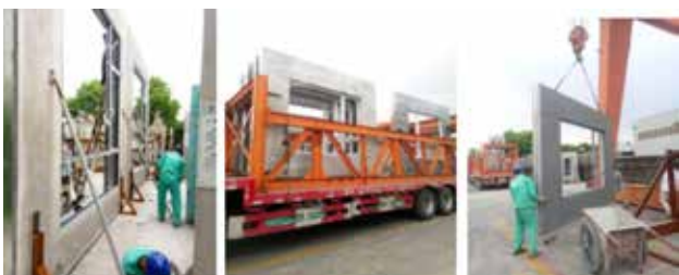
Picture4 Prefabricated external wall lifting site
