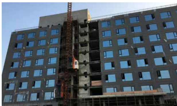
Picture5 Prefabricated external wall construction site
