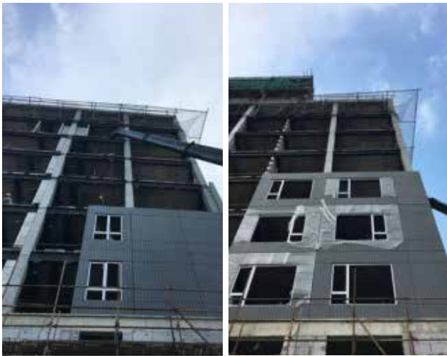
Picture9 Prefabricated external wall construction site
