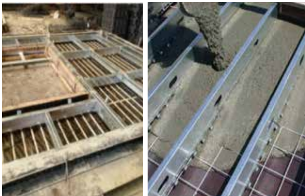
Picture3 Precast exterior wall and window frame
